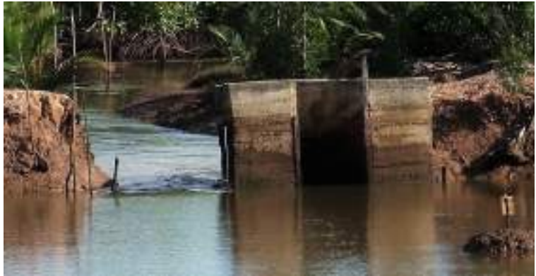
Figure 8: Hydrology is essential to success in restoration. The drainage rate needs to be the same at the restoration site as in the natural mangrove outside the pond. If the channel has a bottleneck at some point (here, the entrance to a former shrimp pond) widen by digging (as done here to the side of the former sluice gate) until drain rates equalize.
