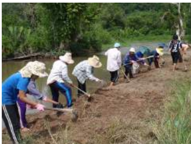
Figure 6: Villagers regrading shrimp pond embankment to increase the area where mangroves will grow. Before this work, the pond had steep walls and a flat, poorly drained bottom. This work produced more area at an elevation suitable for mangrove growth and improved the pond drainage.
